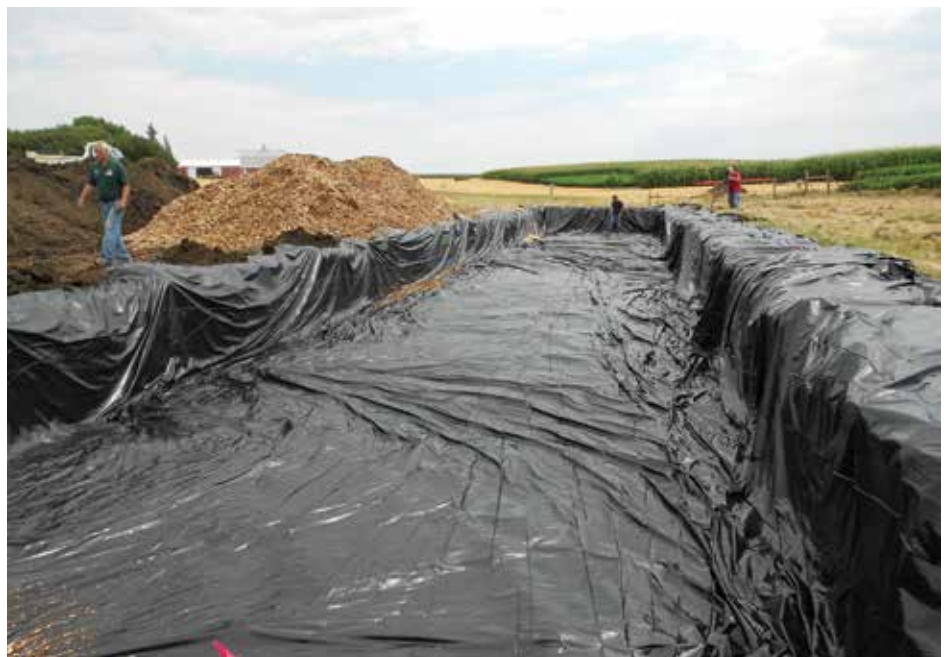
Bioreactor dug, lined, and ready to be filled with woodchips. Image by Chris Hay.
