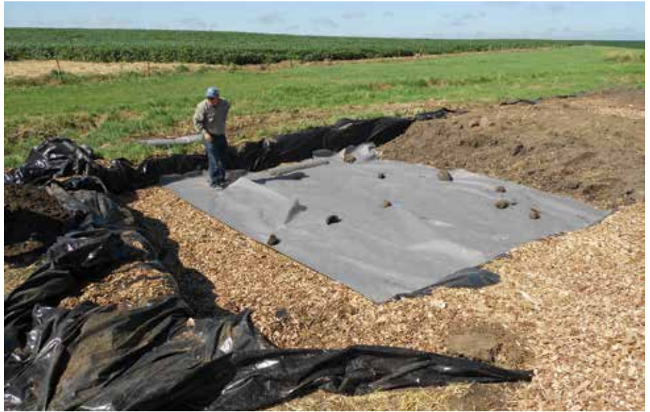
Bioreactor filled with woodchips, geotextile is being laid on top and topsoil is being backfilled onto geotextile. Image by Chris Hay.
